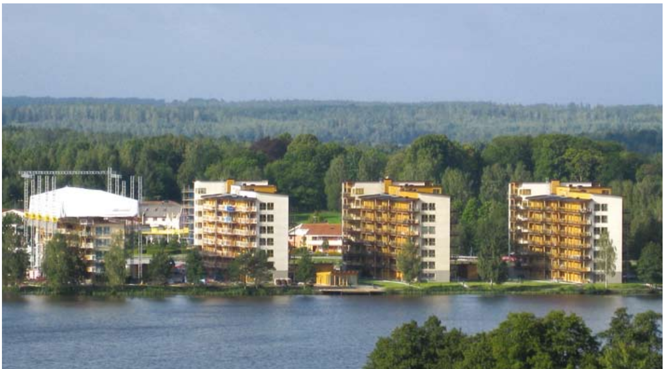
The Limnologen buildings, eight-storey apartment buildings in Växjö, Sweden made with wood structural frames.
